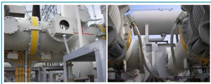
內置型傳感器(Internal Sensor) 外置型傳感器(External Sensor)
